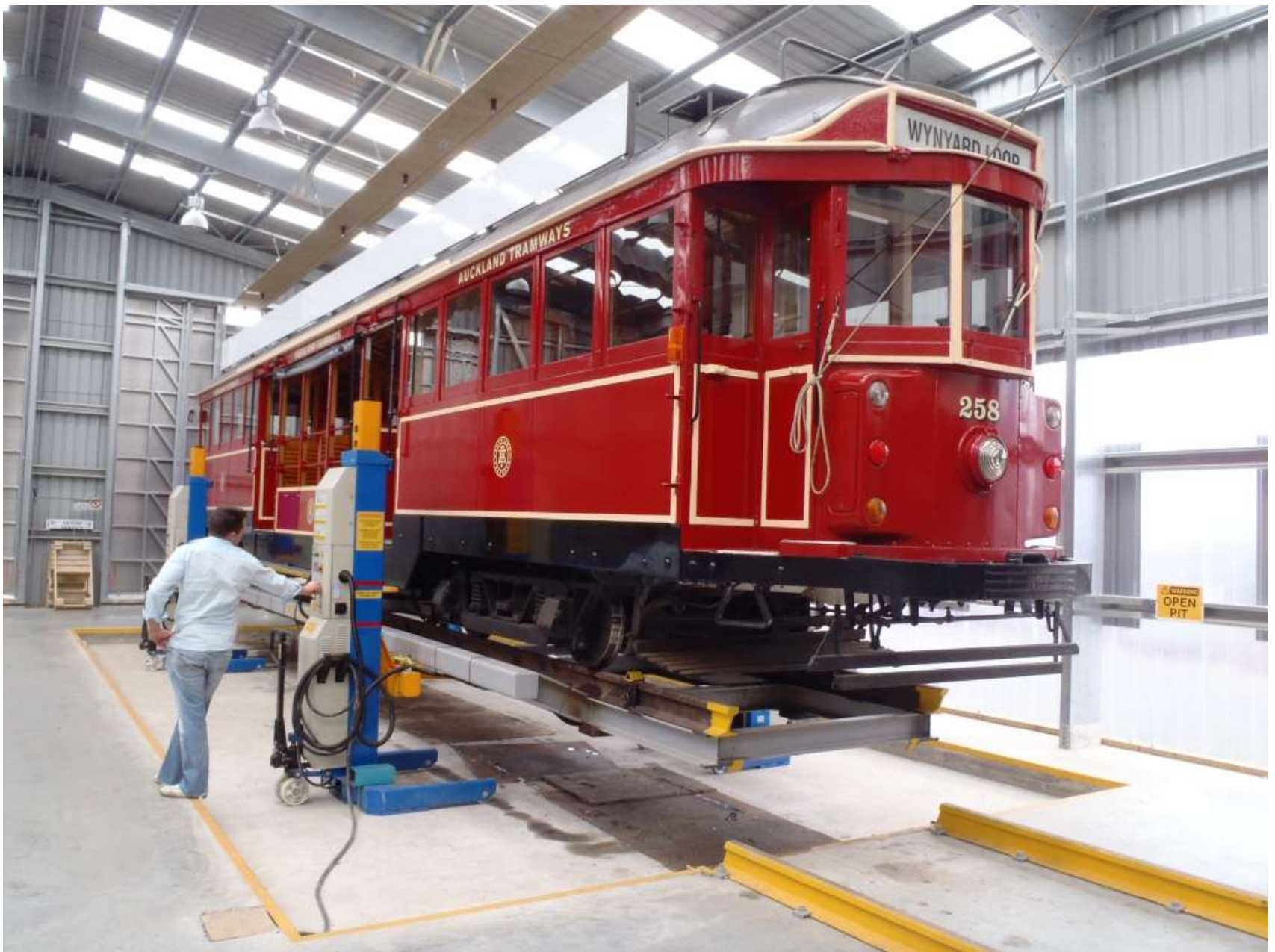
Temporary tram shed with hoist rather than pit
