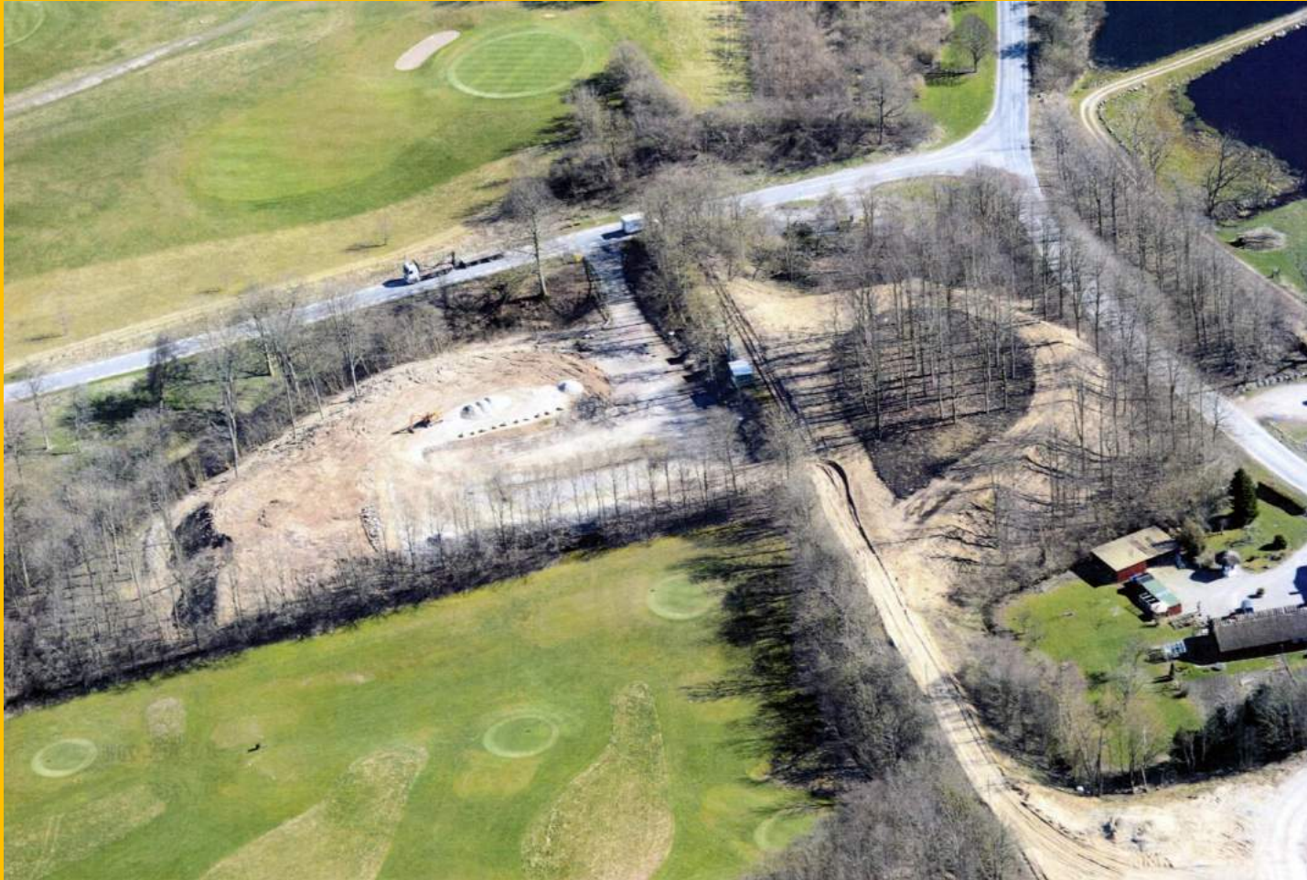
Metre gauge line loop
